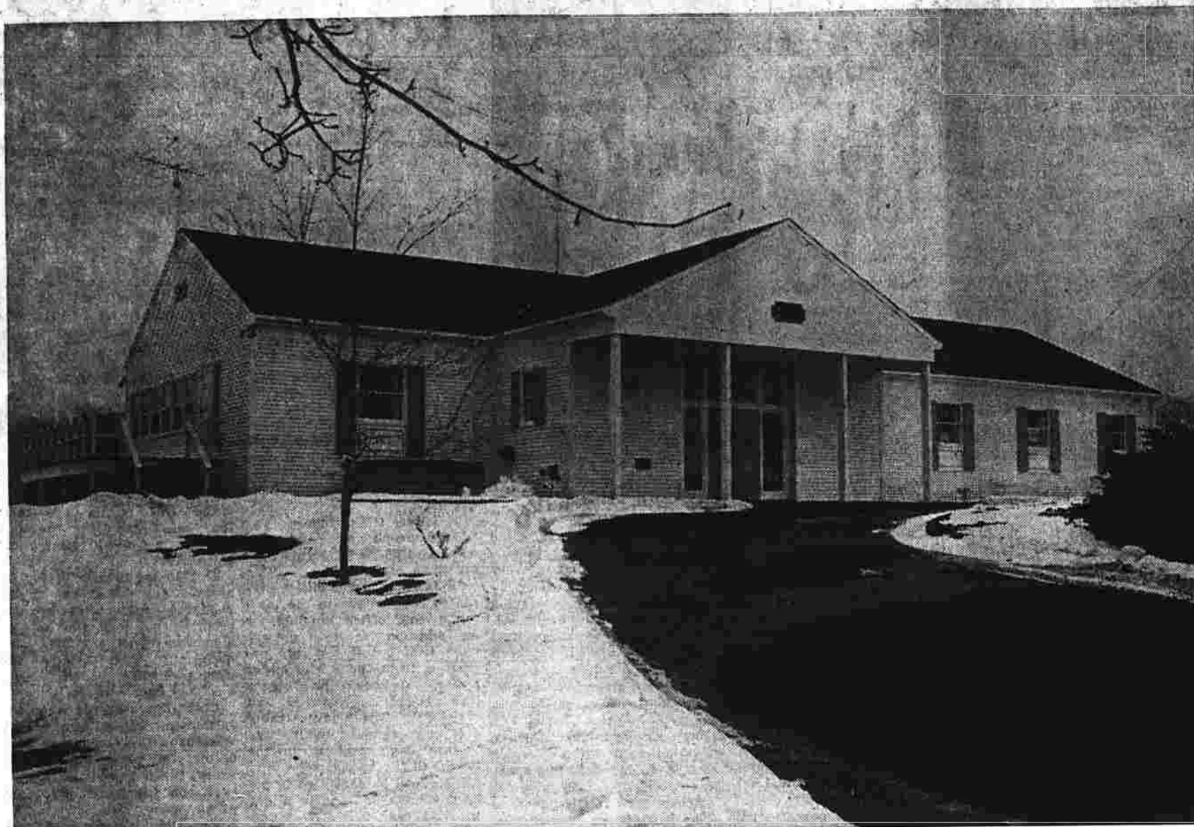
Circular driveway from S. Main St. leads to Colonial portico entrance of Manchester Country Club's new building.
