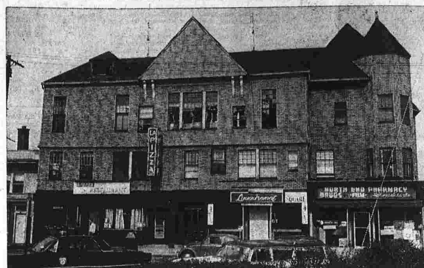
Broken windows on the third floor of a large building at 10 Depot Square mark the area from which 12 persons were evacuated during an early morning fire.
