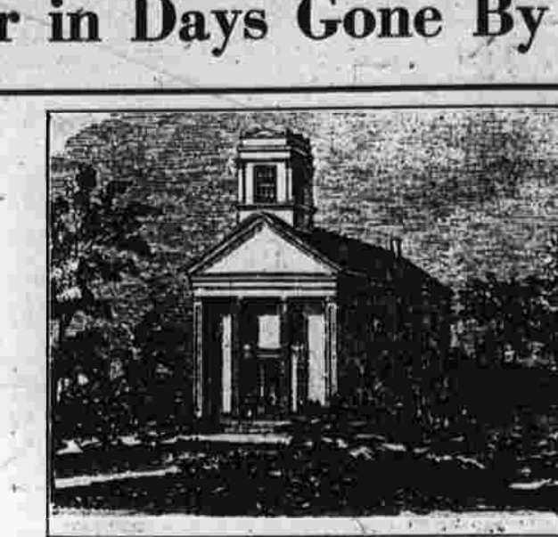
The East Academy, formerly located on Parker St. This structure is typical of the smaller public buildings in the Greek Revival style. It has a pillared front, with a low, square tower with pillars at the corners.
