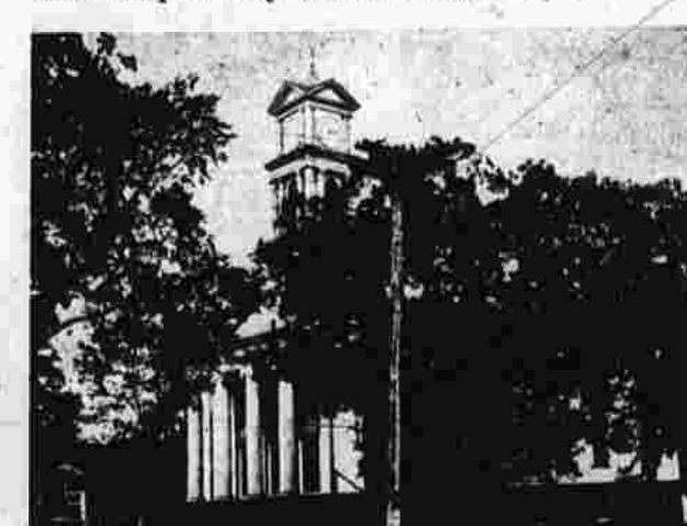
This church was built after 1820, when the Greek revival was in vogue. However, it has a lovely, wide portico of fluted Doric columns at the front and the tower, (removed a few years ago) had the columns and pediments of the Greek revival church.
