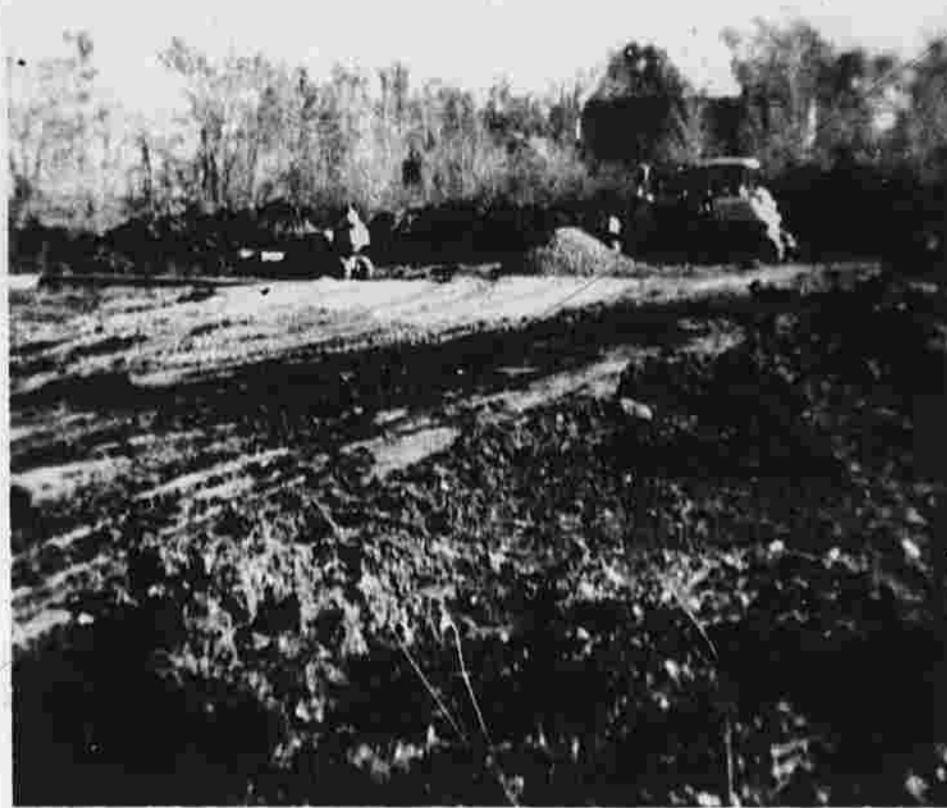
Bolton Library Under Construction
