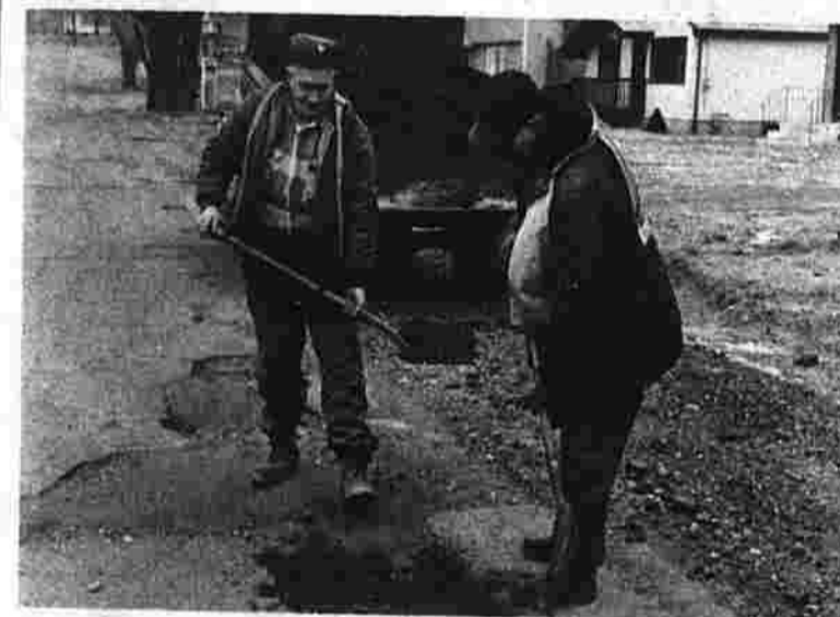
Patching of potholes in roads is a continuing job of the Highway Department when winter or spring thaw plays havoc with the road surfaces.
