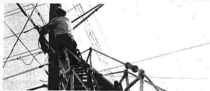
The town's fire alarm system was extended in 1975 with nine new fire alarm boxes installed in the Forest Hills area. Area residents were instructed on the procedure to follow when activating a fire alarm box. The wires for one of the boxes is shown being strung.
