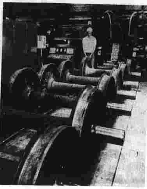
This hard hat may not look like a barber. But his is preparing these freight-car wheels for a shave. He is a late operator who uses a computer to determine how much steel must be shaved off the wheels to restore proper tread contour at the Havelock wheel shop of Burlington Northern.
