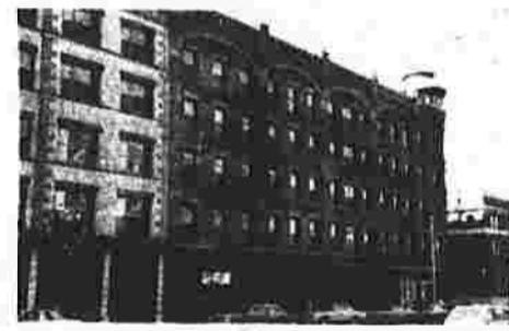
The Linden Hartford — Renovations
