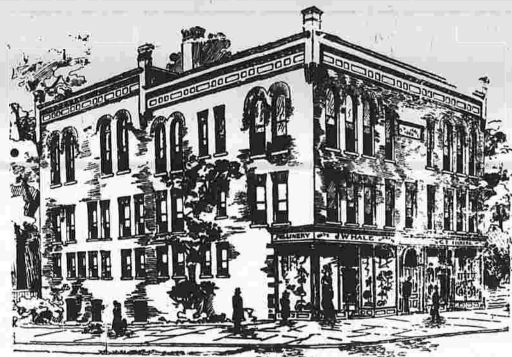
This is an ink drawing for the first House and Hale building at Main and Oak streets. It was built in 1896 and burned down in 1909. A new building replaced it. (Loaned by Charles S. House)
