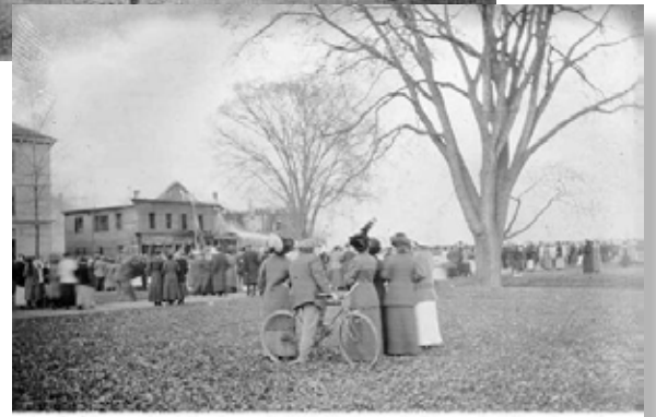
Town's folk watch helplessly as the Pola Store and adjacent buildings burn along the north side of School Street. The 3- story building at the far left is Keith's Furniture Store. To add insult to injury Hose Company #4 was reduced to ashes. The entire 32 room Ninth District schoolhouse was destroyed in a matter of one hour.
