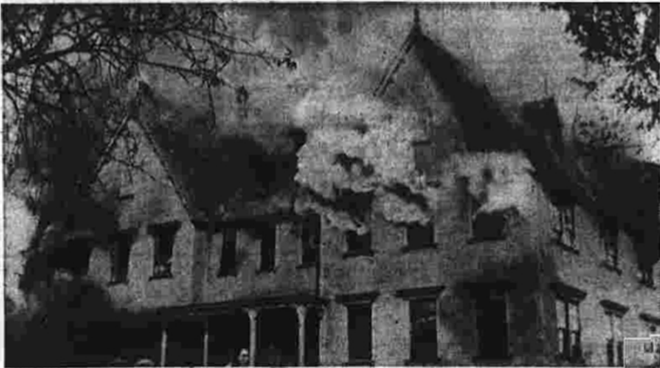
Smoke and flames shoot from the windows at the front of the school.
