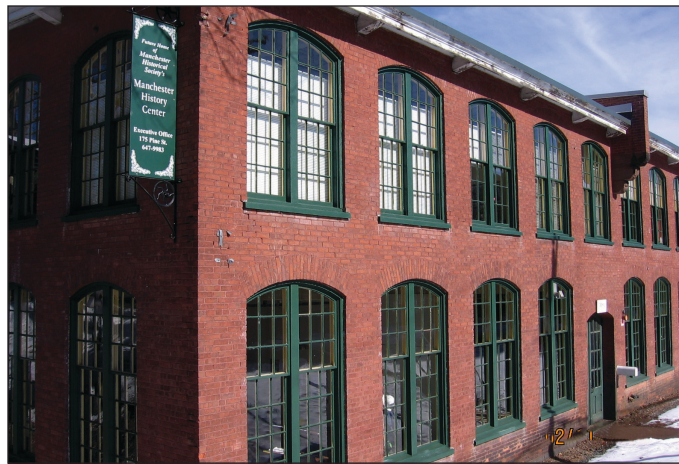
Some of the restored windows at the Manchester History Center.
