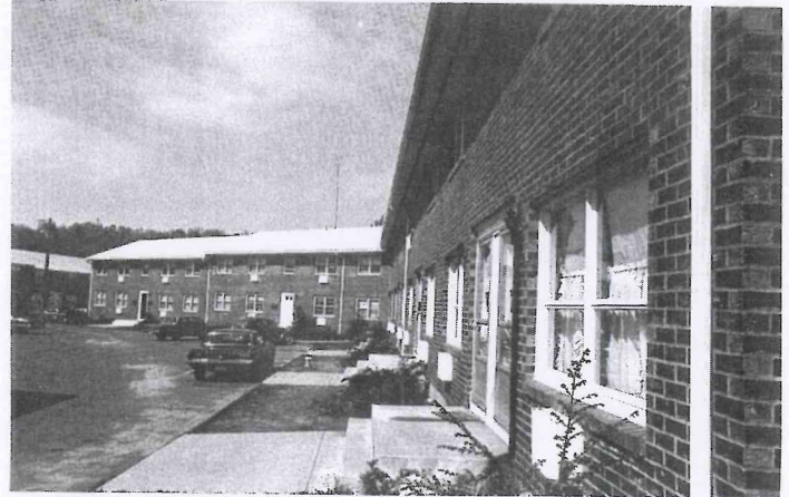
Woodbridge Gardens, Woodbridge Street, Manchester
