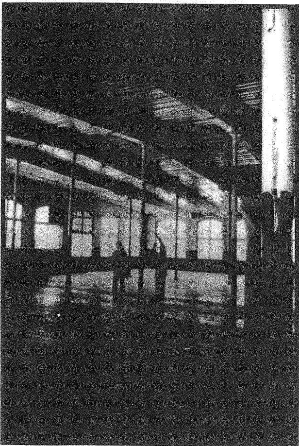
Interior of 210 Pine Street Yarn Mill
