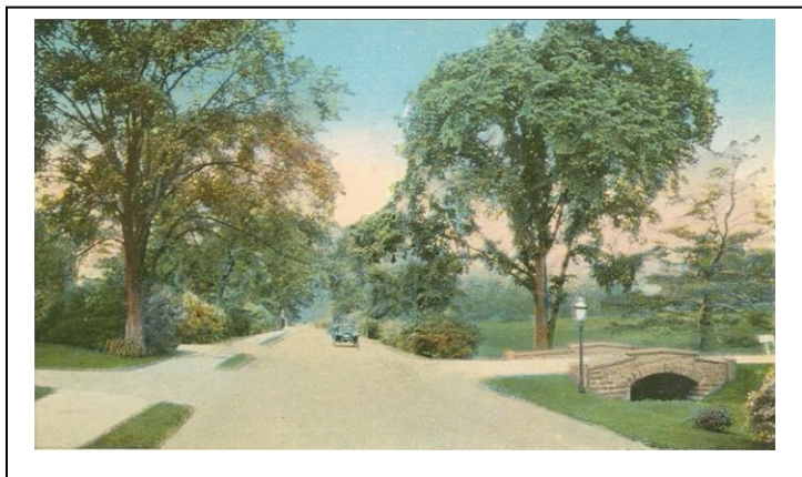
Left: Early 1900s postcard shows Hartford Road with a stone bridge, evidence of the dry brook. The picture was taken near the junction of Main Street and Hartford Road looking west down Hartford Road. The Great Lawn occupies the right side of the scene.
