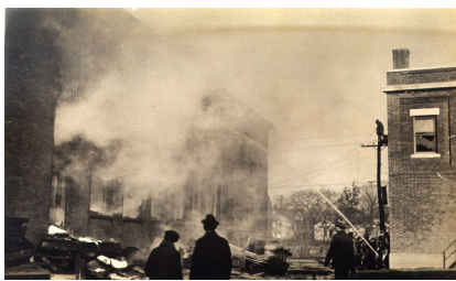
Fire at the Herald's Hilliard St. building, November 18, 1922. Photo by John Knoll. [Webmaster's note February 2016: Fixed up, the building became the home of Able Coil. It is still there, on the south side of Hilliard St. near the intersection with Main St.]
