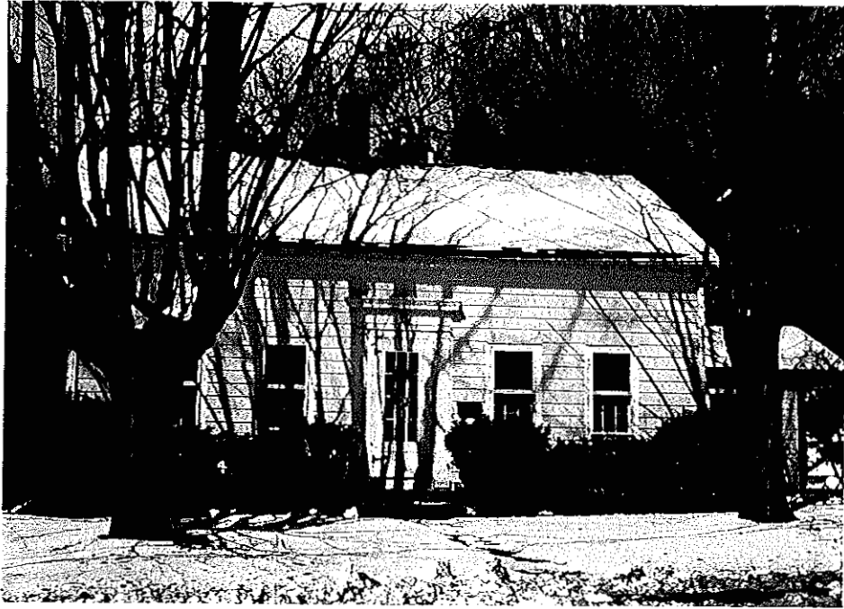
113 Spring Street, Millworker Tenant Housing c. 1840-1850
